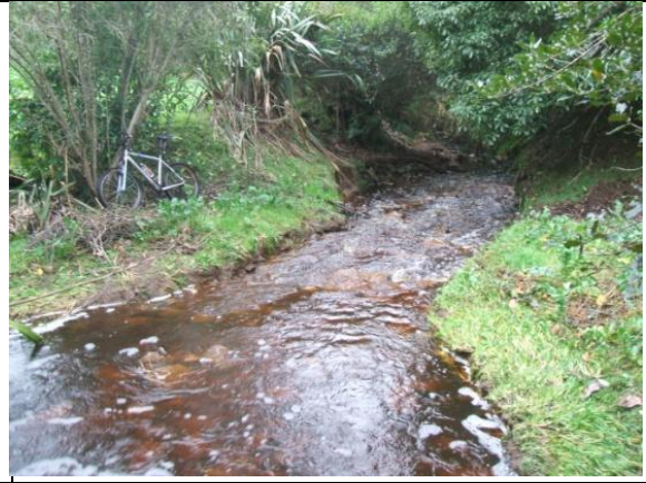
12. Area 'B' – d/stream of culvert
