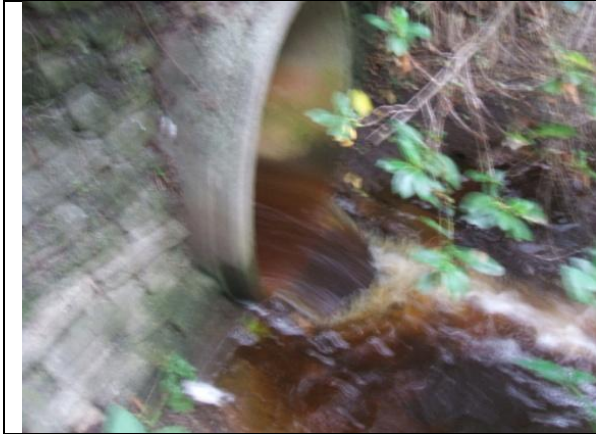
11. Area 'B' - John Webb Drive road culvert
